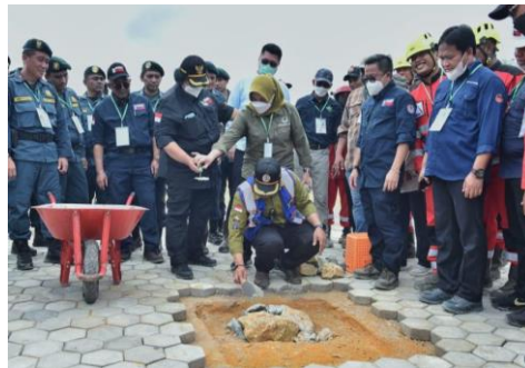
The ceremony of laying the first stone with Ibu Siti Nurbaya Bakar, Minister of Environment and Forestry.
