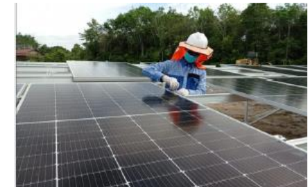
Solar panel installation
